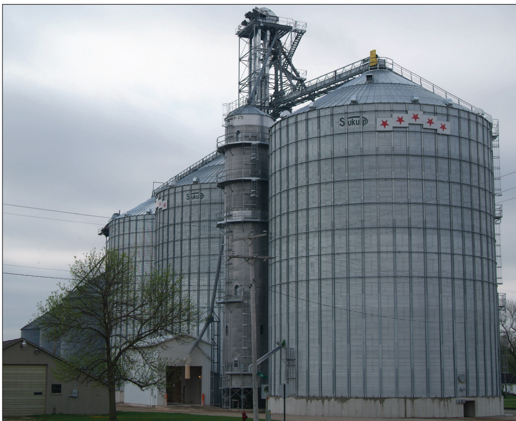
Five Star Cooperative's new steel annex in Hanlontown, IA includes more than 1 million bushels worth of steel storage plus drying capacity at 4,700 bph. Photos by Ed Zdrojewski.
