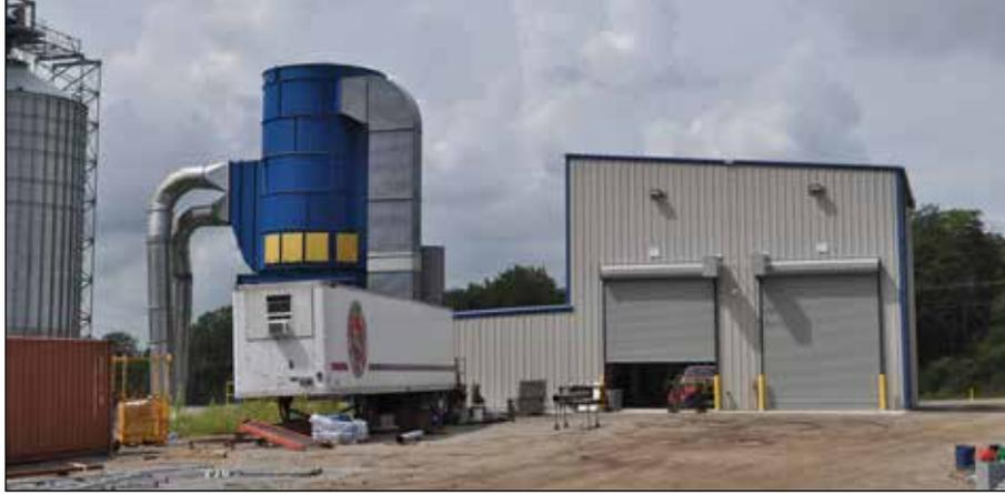
*Twin 1,000-bushel mechanical receiving pits with an AIRLANCO baghouse dust control system designed for use in an urban environment.*
