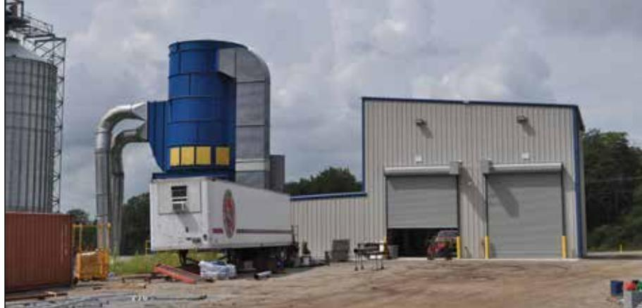
*Twin 1,000-bushel mechanical receiving pits with an AIRLANCO baghouse dust control system designed for use in an urban environment.*
