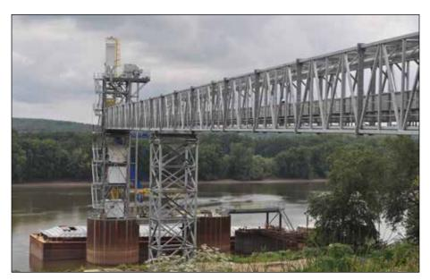
Barge loading station on the Illinois River serviced by a 40,000-bph InterSystems belt conveyor and a movable Premier loadout spout. Photos by Ed Zdrojewski.
